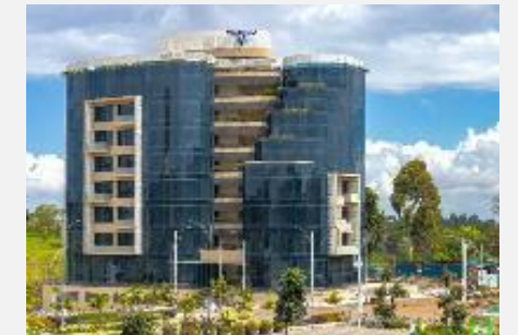
Victoria Commercial Bank- Completed, ready for occupation 14,500 sqm Grade A office
